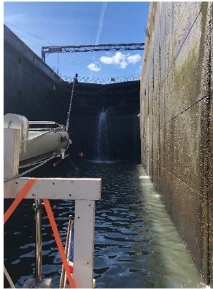
Photo 1: Traditional lock with gates.
